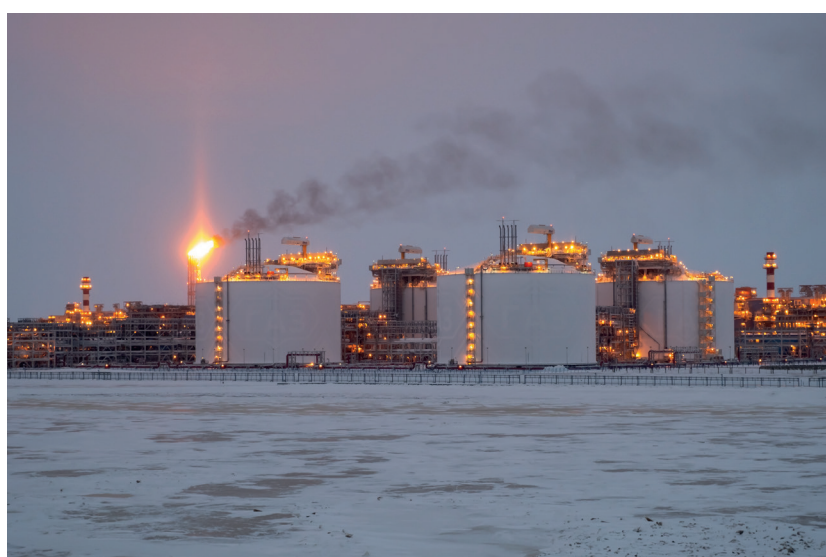
Natural gas processing plant in Sabetta, Russia (Yamal LNG plant). Photo: iStock KadnikovValerij
