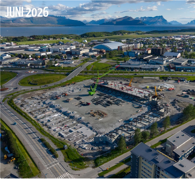
Construction site for Arctic Arena in Bodø, by Ny Arena. Construction sector is the most attractive for entrepreneurs
